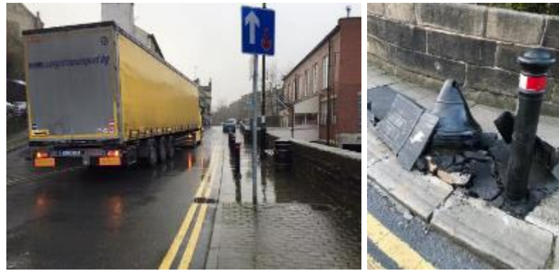
Figure 33 - Truck stuck on Hollowgate, Holmfirth & HGV damage to 'bell' protecting bridge on Hollowgate
