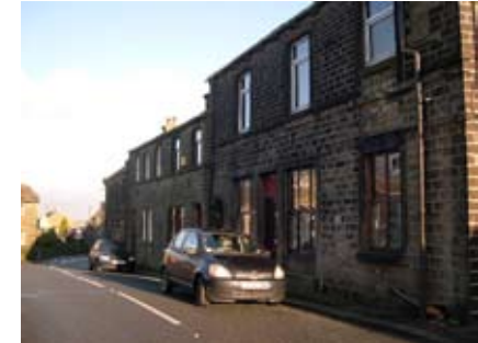
Cottages along Woodhead Road displaying good frontages
