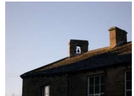
Roof of the Sunday School
