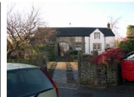
Barn conversion on Woodhead Road
