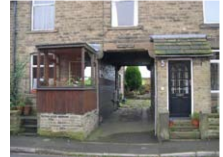
Piecemeal alterations along Bank Lane
