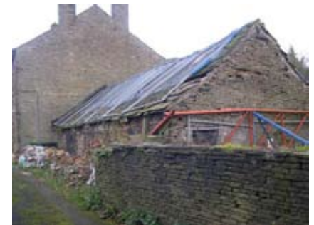
Stone building along Bank Lane
