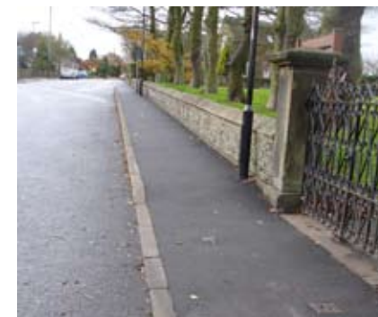
Natural stone kerbs outside the church
