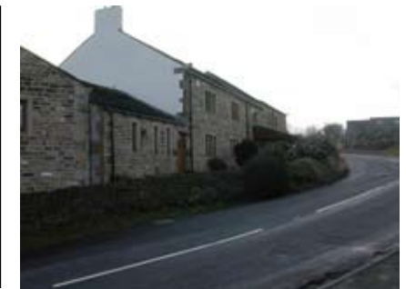
The converted Denroyd Farm
