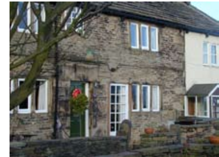
Grade II listed building within the conservation area
