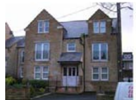
Photo 55. View of modern infill development on Regent Road
