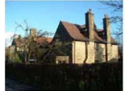
Photo 74. Development along West Avenue
