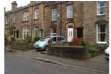
Photo 63. Loss of boundary wall and garden area along Cleveland Road
