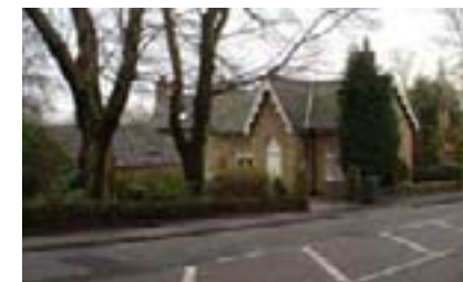
Photo 25. View of the former Lodge to No. 6 Halifax road
