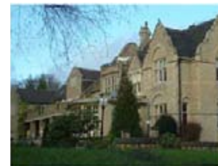
Photo 12. Rear extension to stoneleigh on Bryan Road
