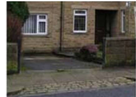
Photo 61. Example of stone sett cross-over along Rumbold Road
