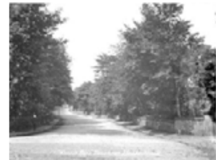
Photo 6. View of Kaffir Rd 1910
