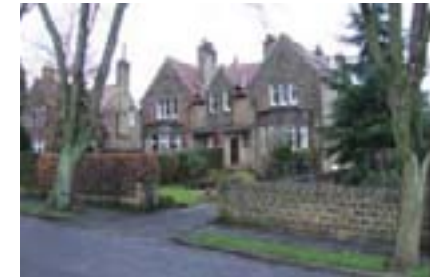
Photo 16. View of the early twentieth century development along the tree lined Talbot Avenue
