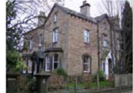
Photo 51. Property on the north side of Imperial Road
