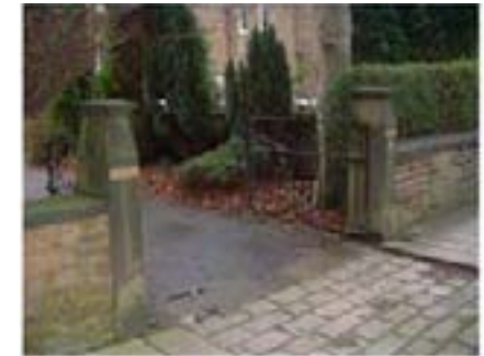
Photo 67. Elaborate gate piers on the south side of Thornhill Road
