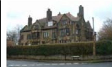
Photo 66. View of a large house on the south side of Sunnybank Road
