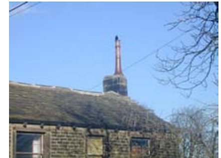
Traditional roofing material found within the conservation area
