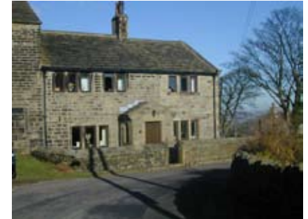
Property within the Upper Oldfield identity area
