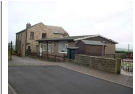
Unattractive pre-fab building
