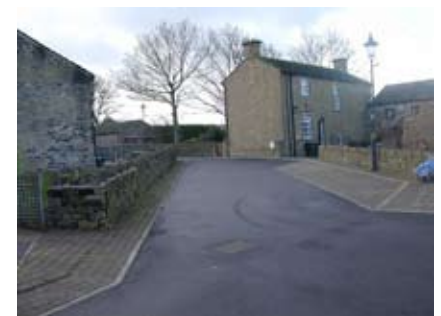
Unattractive floor materials along Balk Lane
