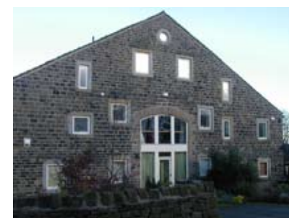
Barn conversion Balk Lane
