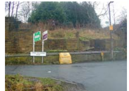
Walls and area on Lower Wellhouse Road
