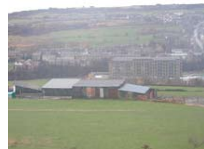
View of Lowest Mill
