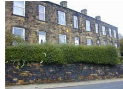
Walls along High Street
