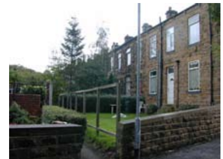
Dwellings at Industrial Avenue
