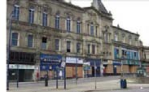
The boarded up shopfronts give an obvious signal of dereliction to the area. The active re-use of this building is a prerequisite for the overall enhancement of Northgate. There is great scope to improve the area by a reduction in the highway dominated character of the space and the incorporation of a more shared-surface treatment and the better accommodation of pedestrian movement across the area.
