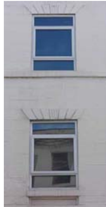
Painted stone walls and replacement pvc windows completely change the character of the building
