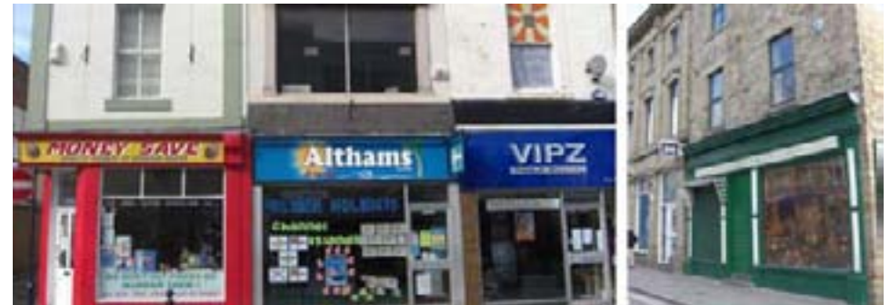
Examples of shop fronts on Westgate that detract from the quality of the buildings compared with a more sensitive period design - even with the inclusion of shutters.
