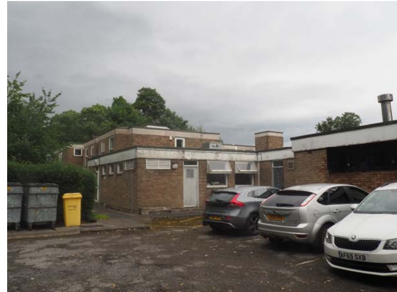
Existing Knowl Park House building (rear car park)
