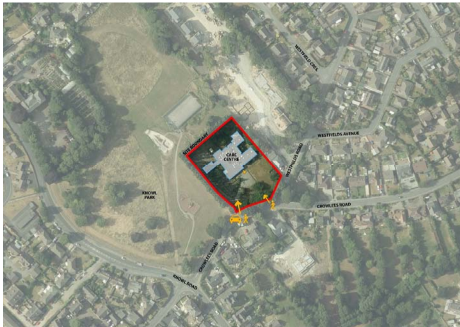
Existing site aerial image
