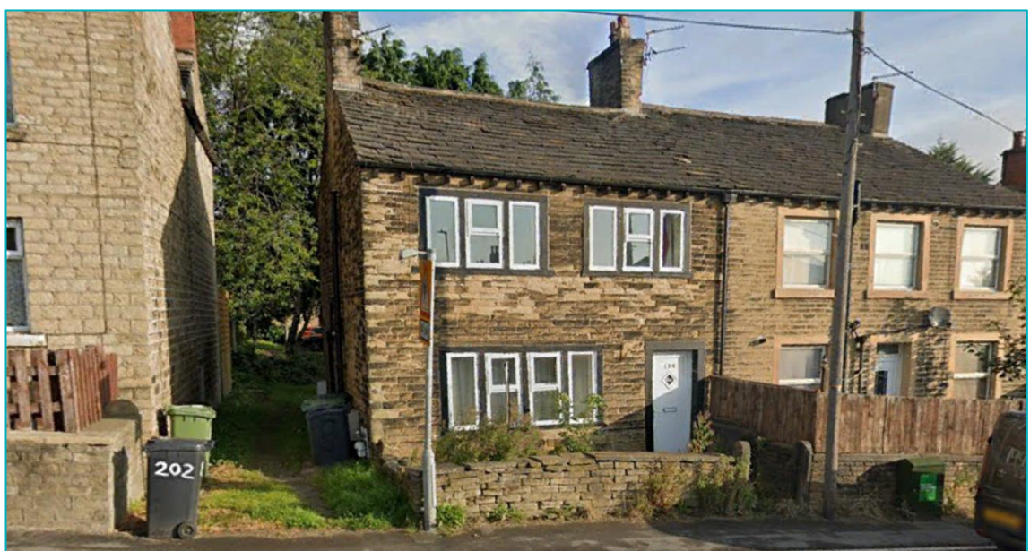
Figure 4.2 194 – 200 Blackmoorfoot Road (Grade II)
