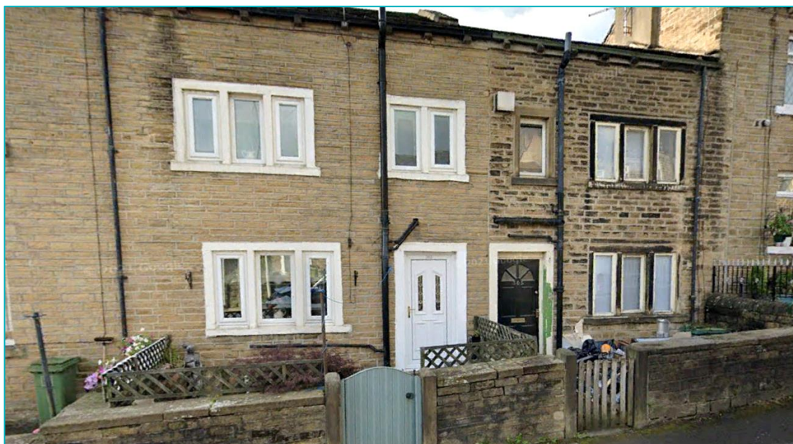
Figure 4.3 303 and 305 Blackmoorfoot Road (Grade II)
