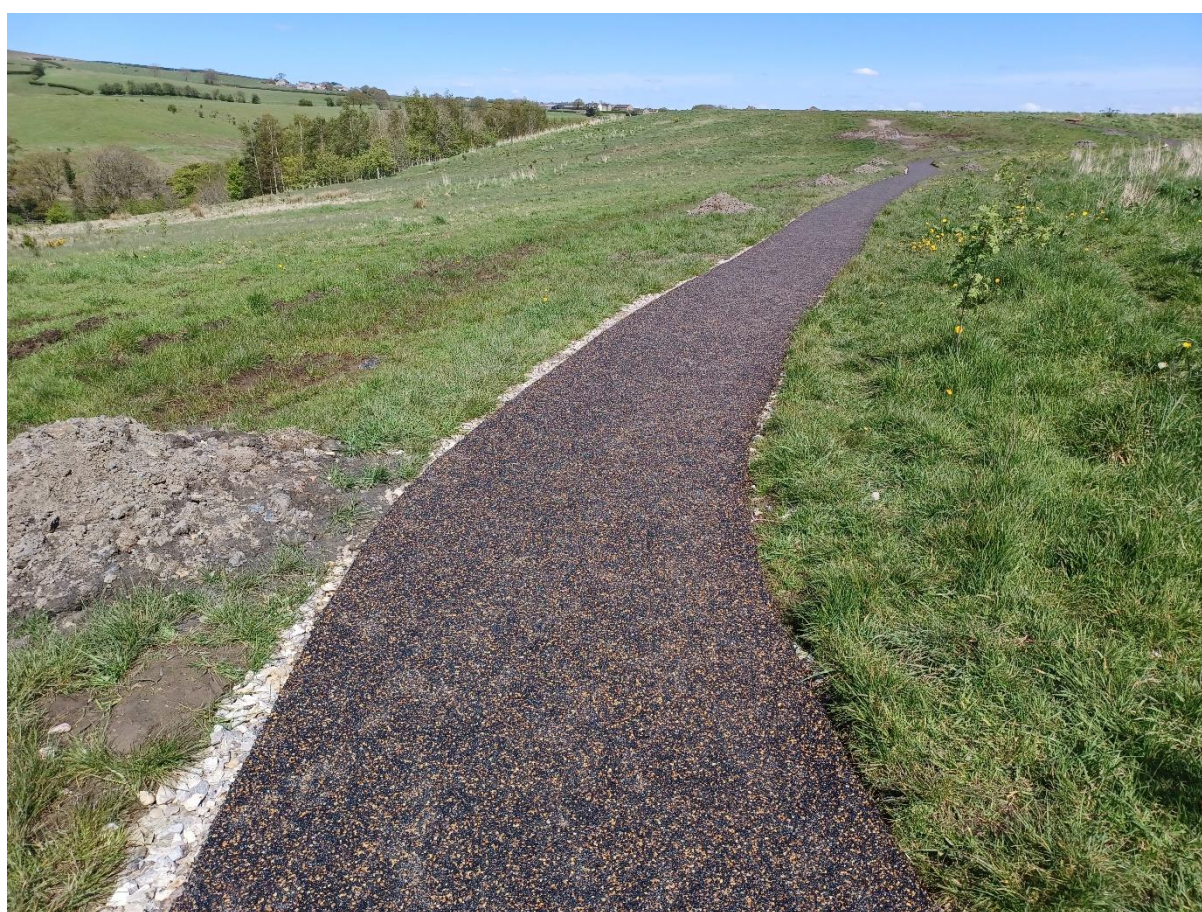
Improved recreation facilities at Park Gate, Skelmanthorpe
