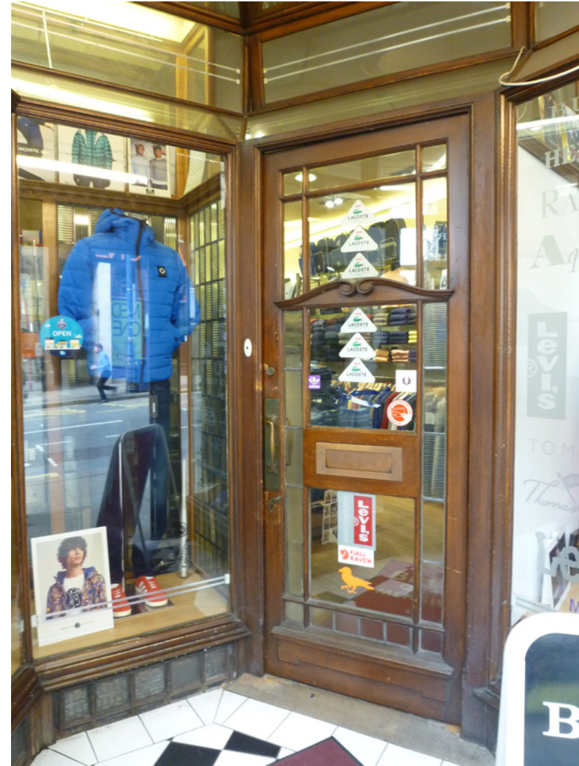
Recessed doorway with an historic glazed, panelled door
