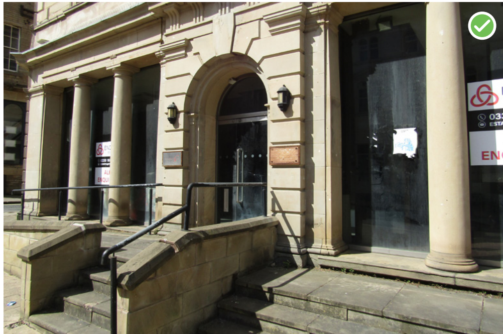
A ramp has been installed adjacent to the stairs of this property on Northumberland Street. In some cases this may not be practical or appropriate due to pavement width or the external appearance of the historic building.
