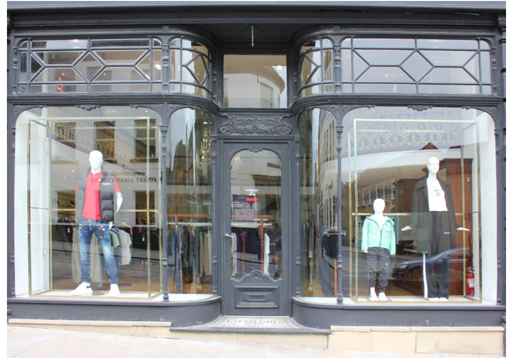
High quality late 19th / early 20th century shopfront on Westgate.
