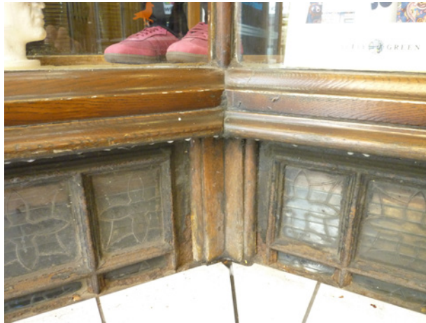
A timber and glazed stallriser on 5 Westgate
