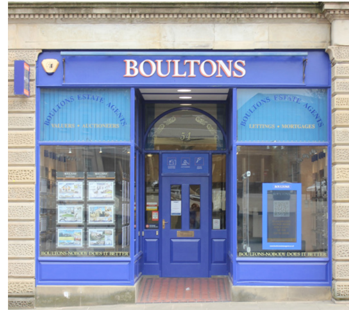
A restored traditional shopfront on the Lion Buildings, John William Street. Transoms divide up the shop windows, whilst the stallriser and fascia are of modest height giving an overall balance to the shopfront. The stone pilasters and continuous entablature are an integral part of the building's façade.
