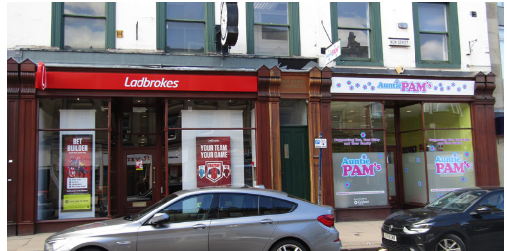
A row of well proportioned, modern but traditionally styled shopfronts in the Grade II Listed building along Market Place
