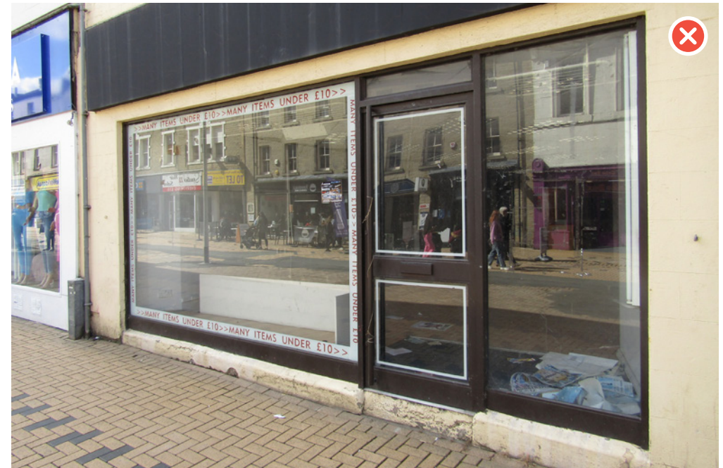
This modern shopfront in a historic building has an unnecessary external step and could easily accommodate step-free access via re-design or an internal sloped floor.
